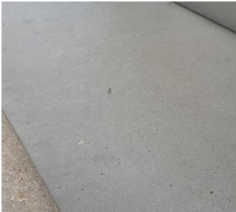
Figure 12. Concrete slab for BPT testing.
